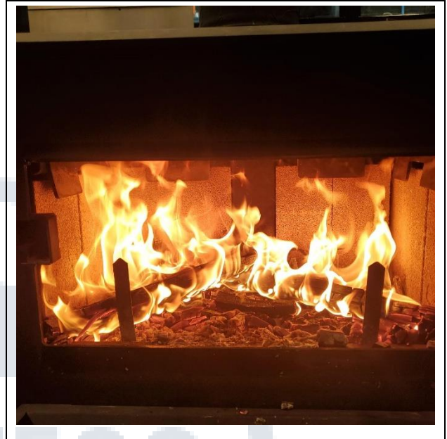
Residual Start-up Fuel Coal Bed – Post Rake
