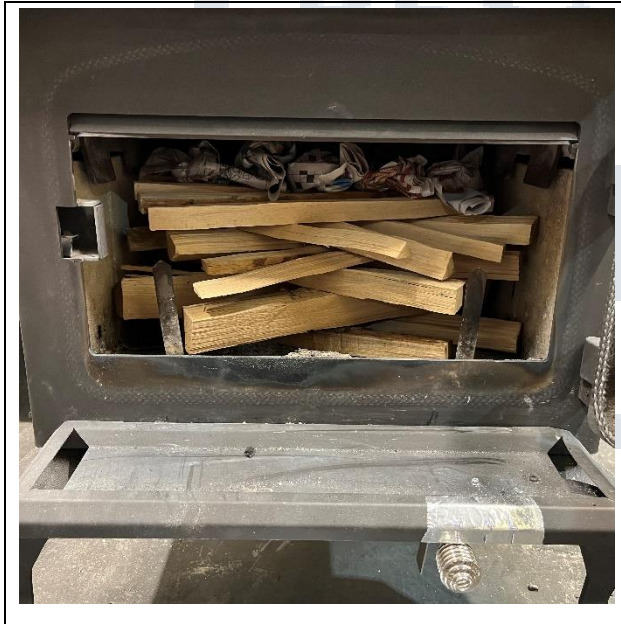
Kindling & Start-up Loaded in Stove
