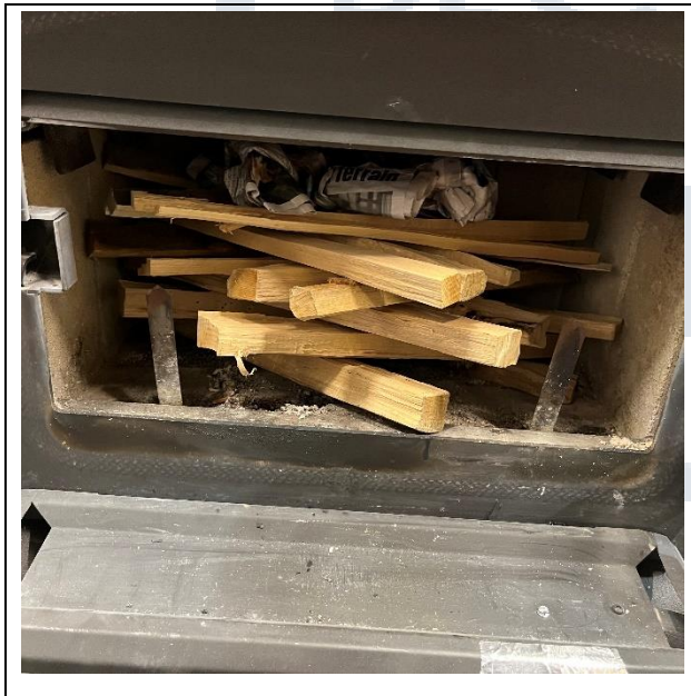
Kindling & Start-up Loaded in Stove
