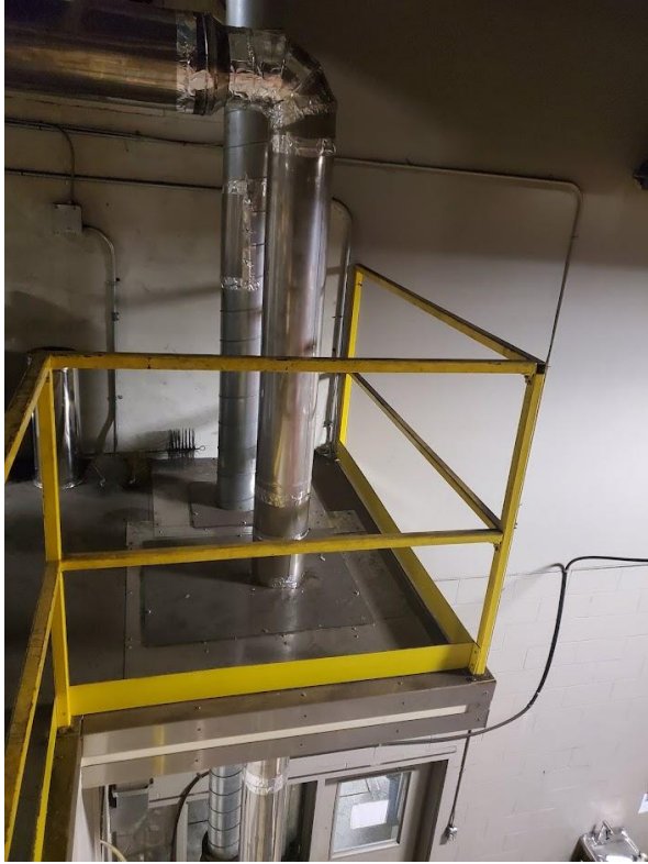
Sampling Section (elbow to floor)
